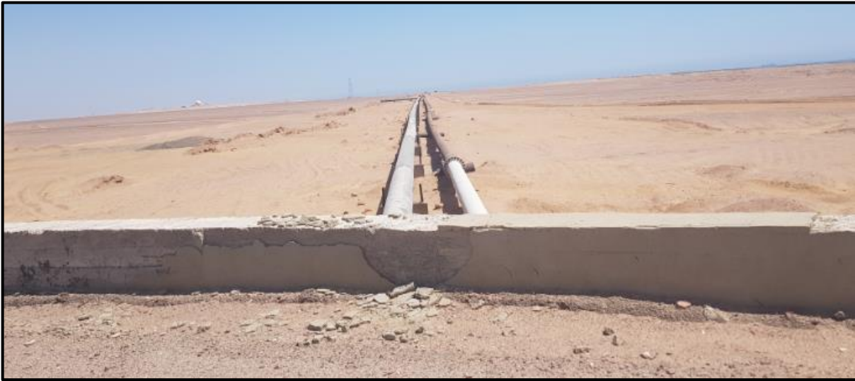
Figure 19: Oil Pipeline East of the Project Site
